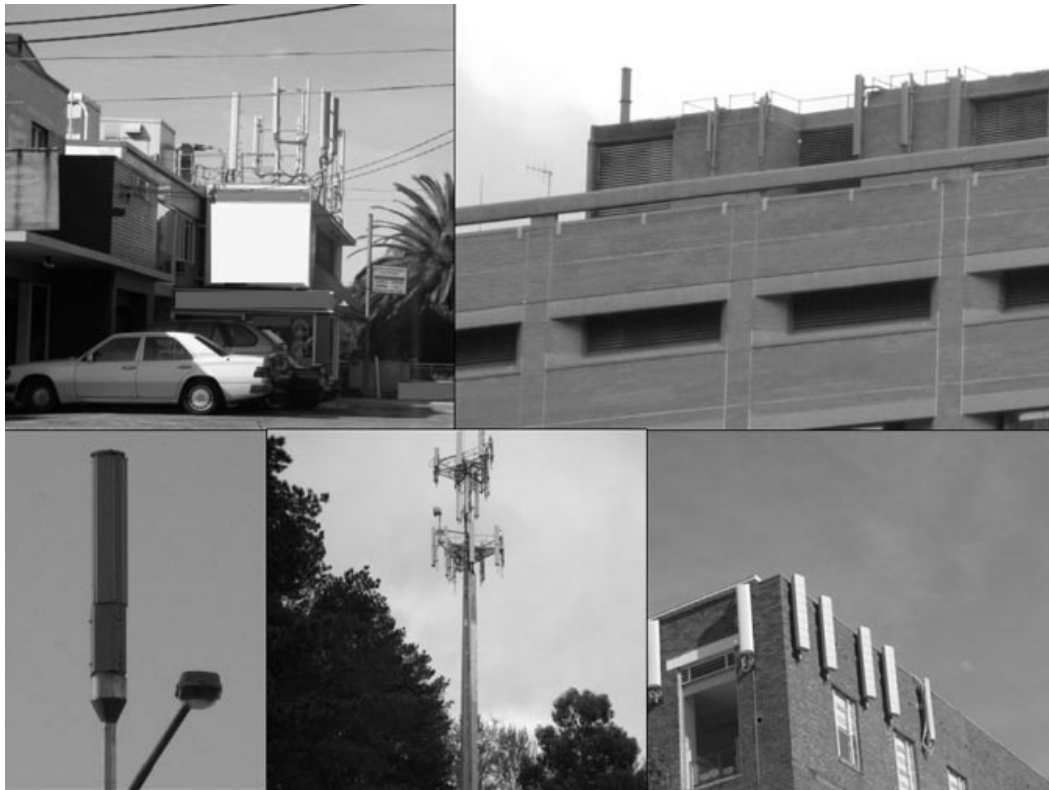
Figure 1—Mobile phone base stations ("antennae" or "masts") in Australia. Upper left: Community shop roof showing plethora of flat panel antennae. Upper right: Hospital roof with flat panel antennae painted to blend in. Lower left: Top of a street light pole. Lower center: Mast erected next to a daycare center. Lower right: Antennae mounted on an office block top floor.
